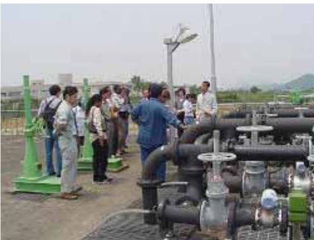
Photo: Training at a wastewater treatment plant
