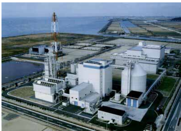
Photo: View of Omuta RDF-based Power Plant
