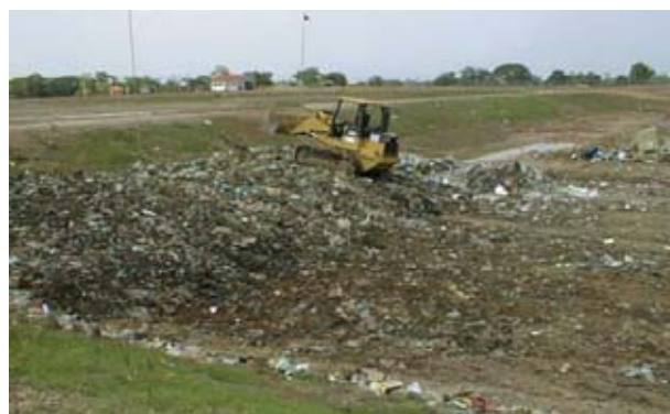
Waste Compaction at the Landfill using Heavy Machinery Granted by the Government of Japan
