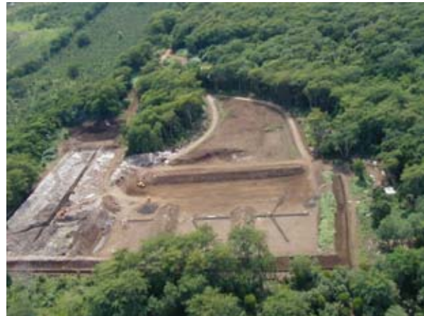
A big rubbish bin under rehabilitation
