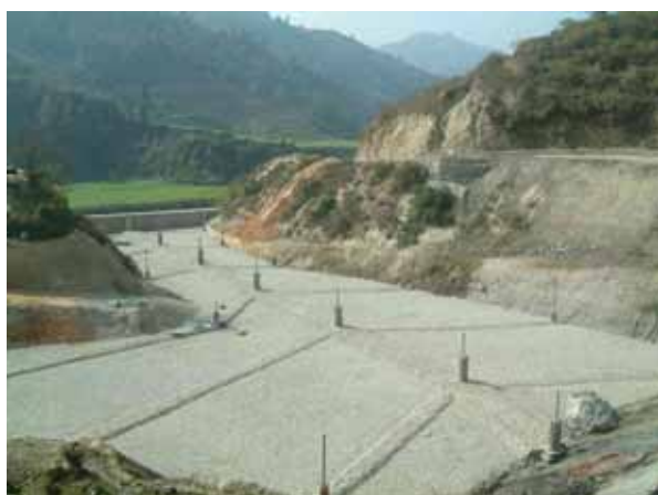
Photo: Sisdol landfill improved as a semi-aerobic system under the pilot project of the Study
