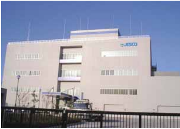
JESCO's Tokyo PCB Waste Treatment Facility
