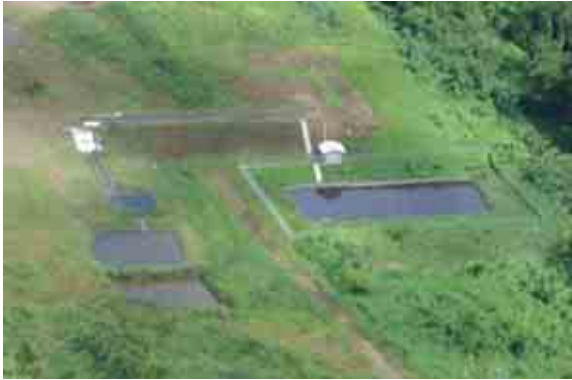
Aerial shoot of leachate treatment facilities
